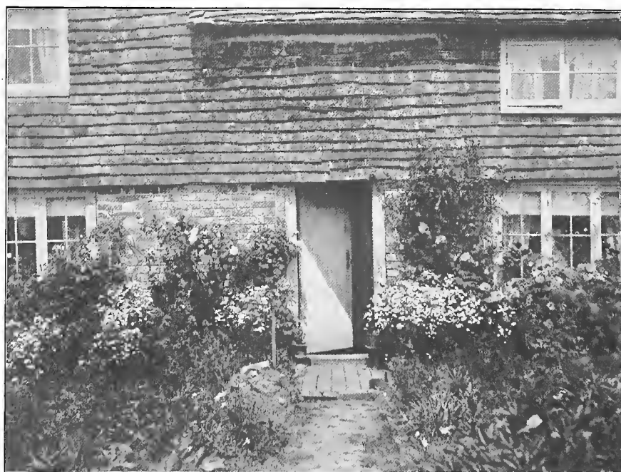
A TILED HOUSE AT BROOMHAM, SUSSEX
